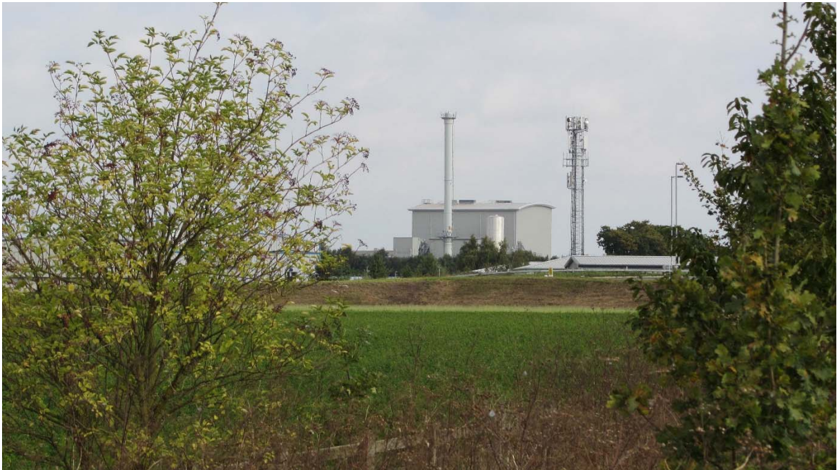
Boiler with stack
