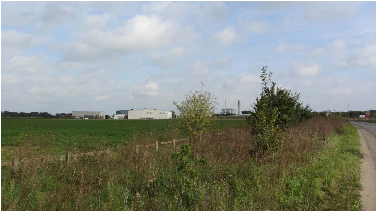
Plant as seen from the adjacent road.
