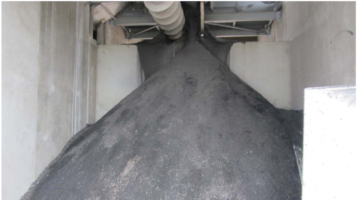
Ash pile at bottom of the boiler
