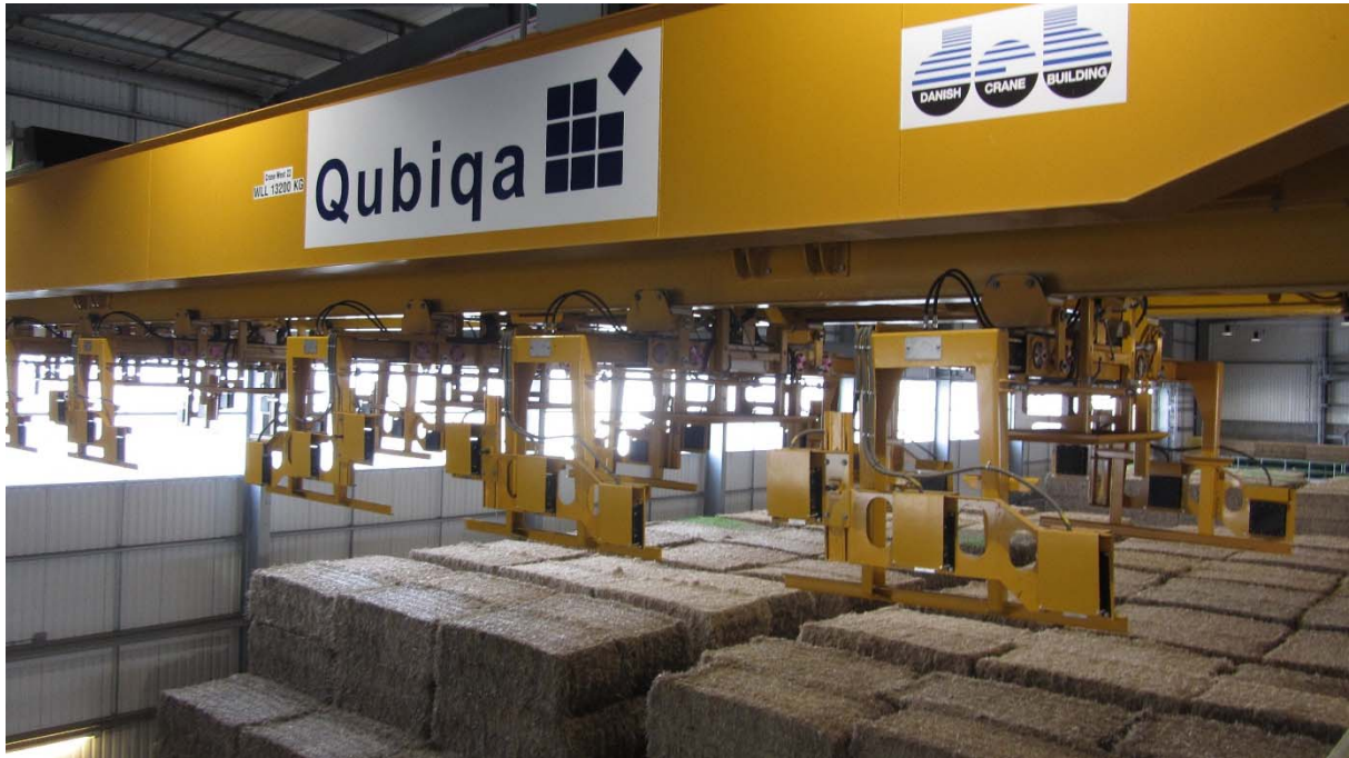
Straw unloading crane.
